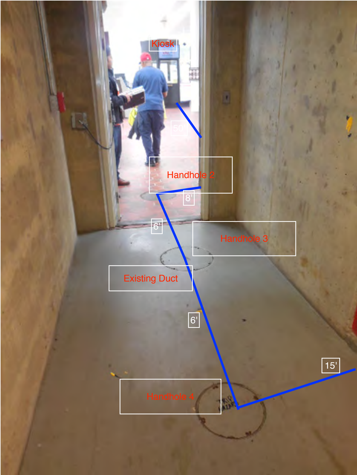
Photo#3 – Existing duct layout in back room corridor
