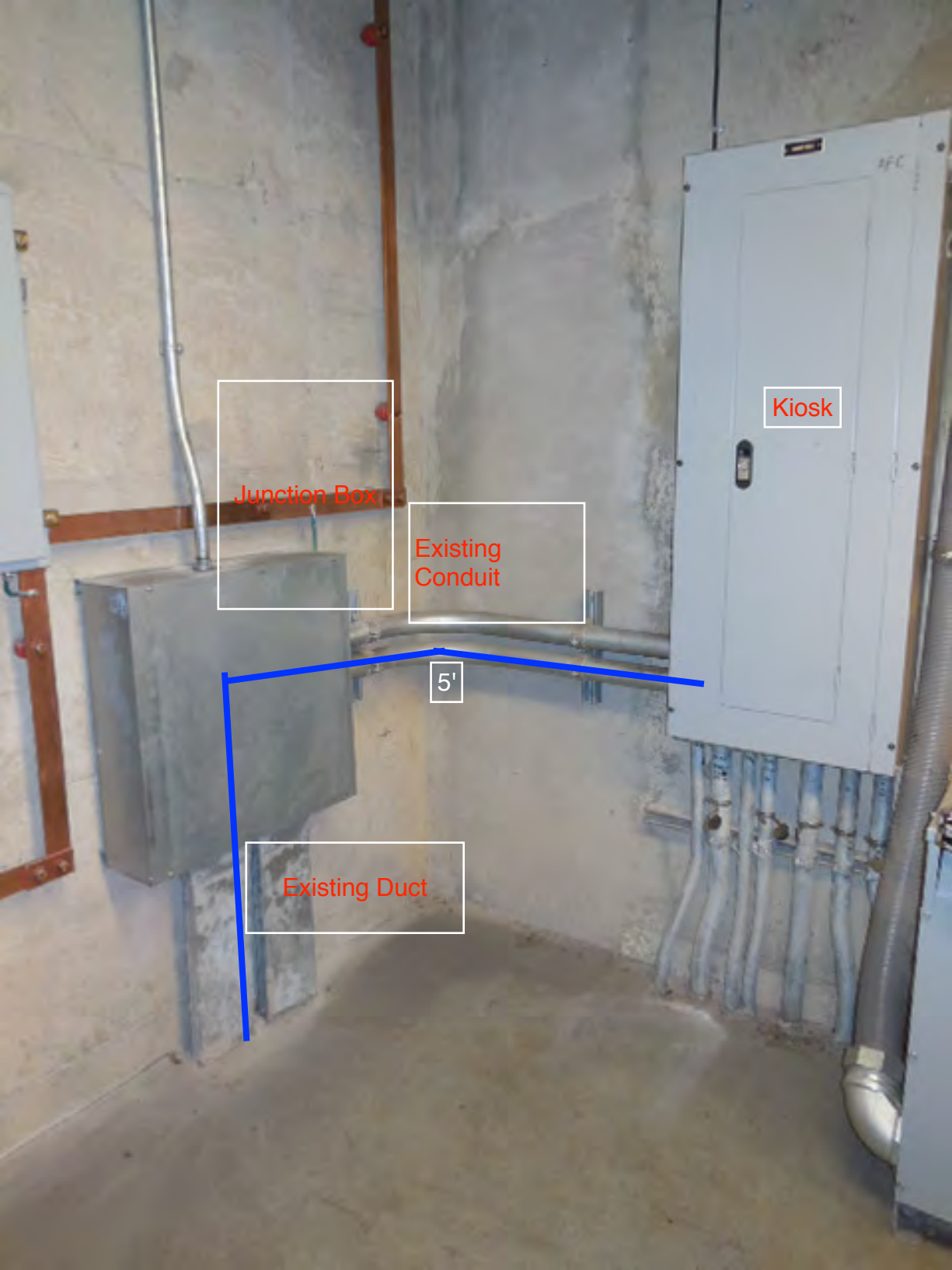
Photo#4 – Existing duct and conduit layout in Room 205
